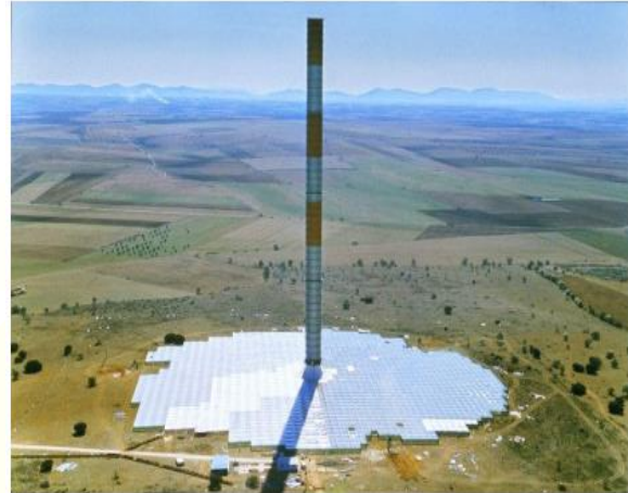
Fig.1. Proto-type Solar Tower in Manzanares, Spain
